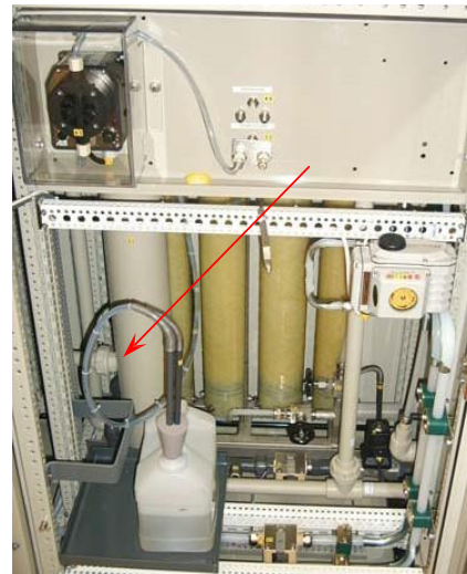
Inlet connection to low side port
